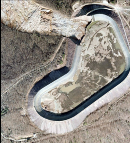
Orthoimagery of failed Taum Sauk Reservoir
