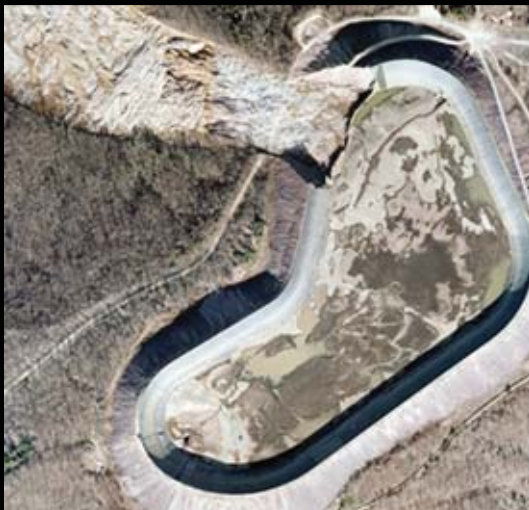
Orthoimagery of failed Taum Sauk Reservoir
